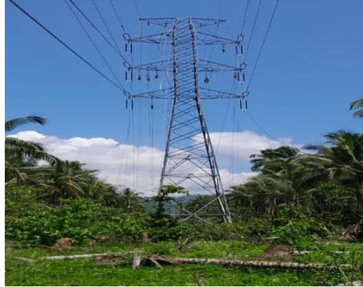
Gambar 2. 6 Tower SUTT 70 kV GI Namlea – GI Namrole
