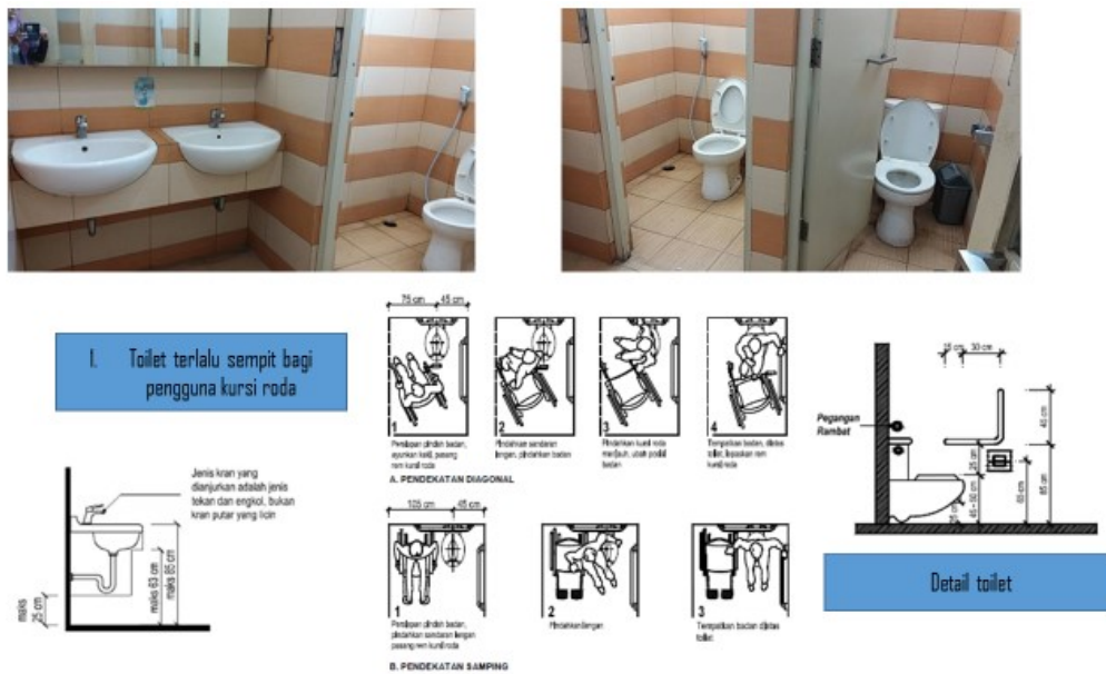
Figure 7. Access to toilets at the Tower building isn't in accordance with universal design principles specifications are difficult to spin for wheelchair users. The proposed design on detail picture of size of toilet.
