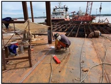
**Fig. 2.** The Welding process for the outer part of the oil cargo tank area
