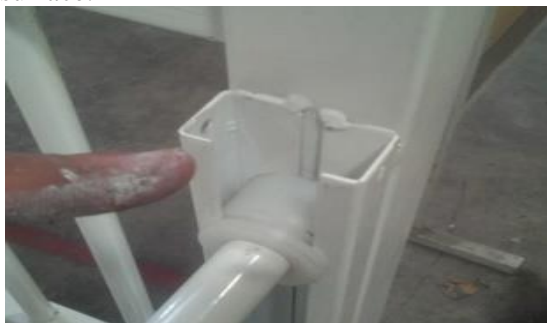
Figure 3. Coating defect
