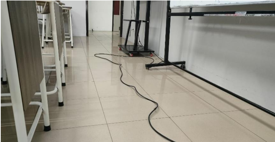
Figure 2. Cables are blocking the path
