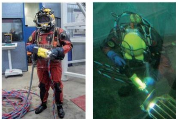
Fig. 6: Underwater treatment process using HFMI/PIT
