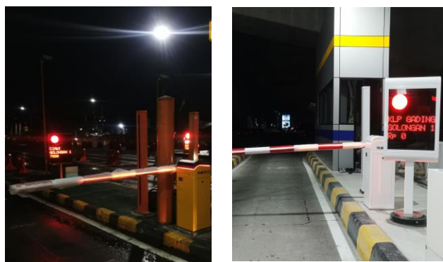
Fig. 12 Trial Unit in toll plaza (a) Ciawi; (b) Kelapa Gading
