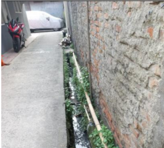
Figure 1. Land Conditions in Narrow Alleys
