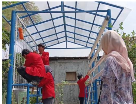
Figure 1. Hydroponic Installation Activities
