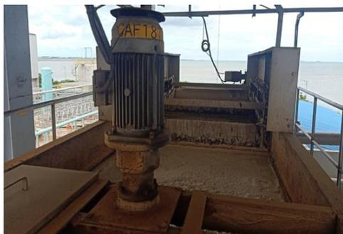
**Gambar 4:** Cavitation Air Flotation (CAF) di PT. X
