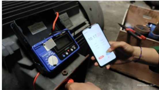
Figure 1. Insulation testing with a megohmmeter
