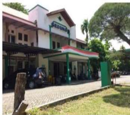
Figure 1. Mechanical Engineering Laboratory, Islamic University of Riau
