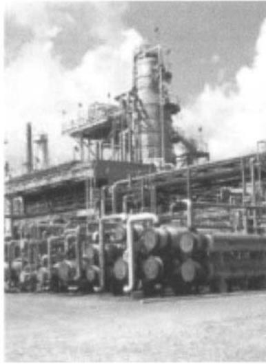
Figure 5–1 A refinery designed to ASME B31.3. (Printed by permission of Bentley Systems Incorporated.)
