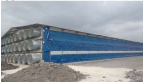
Gambar 2 Kandang ayam sistem tertutup (closed house)
