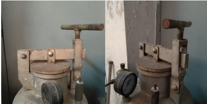
Figure 4. Valve on the acetylene gas
