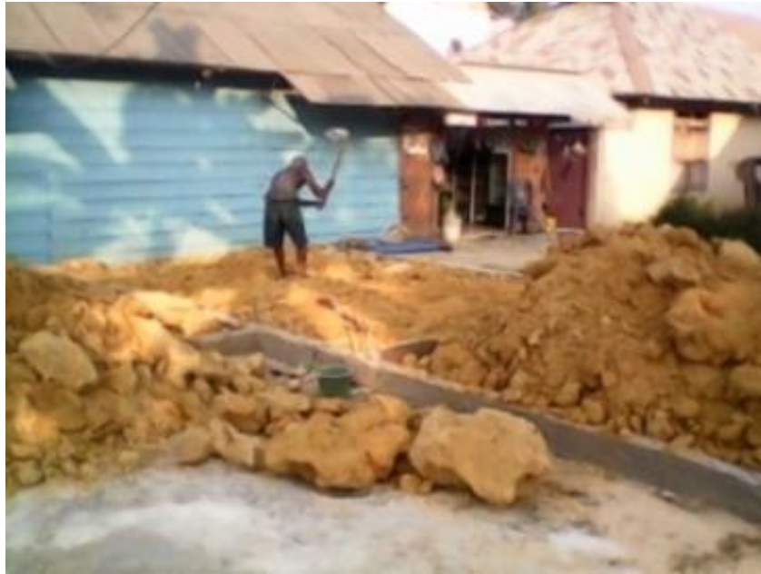
Figure 2. The foundation is stockpiled
