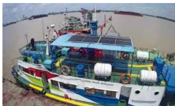
(b) Installed PV Panel
