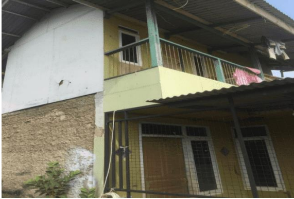
Figure 20. The facade of this two-story house uses brick walls on the ground floor, but the walls on the second floor use GRC (glass fiber reinforced cement) and wood
