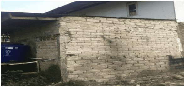
Figure 16. The addition of building mass for toilet and kitchen functions can be seen behind the stilt house with brick walls
