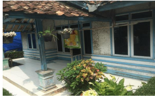
Figure 18. Front view of the stilt house building which has undergone changes to the terrace along the front side with the use of ceramic material as a floor covering, in contrast to the surrounding buildings which use wood
