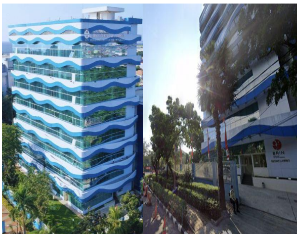
Figure 11. The Front View of The Existing BRIN Building
