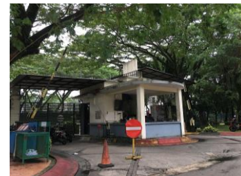
Figure 27. Permeability Location Points (1) in Emerald Residence. Source: Personal Photo
