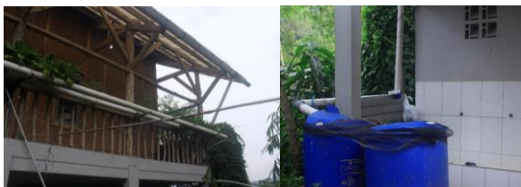
Figure 7. Drums for collecting rain water in the wooden house
