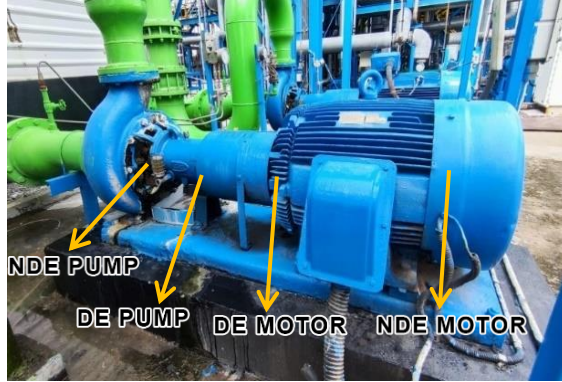
Figure 2. Centrifugal Water Pump
