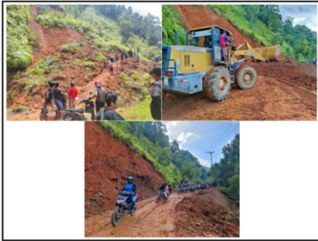
Figure 8. Landslides Disaster in the Road Network Area
