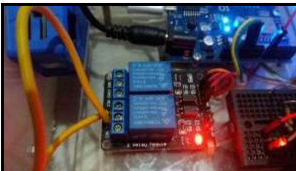
Figure 10.Testing of 2 Channel Relays
