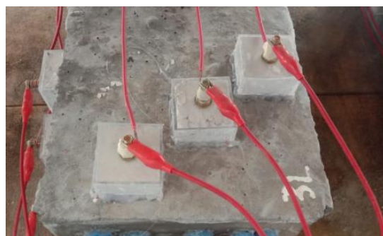
Figure 2. Al-Zn anodes installation
