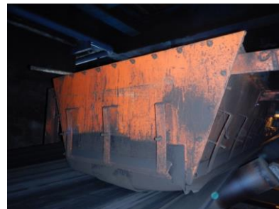
Figure 10. Tailbox extension at transfer point area
