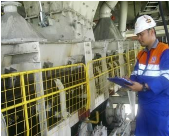
Figure 4. Assessment of coal handling facility by consultant
