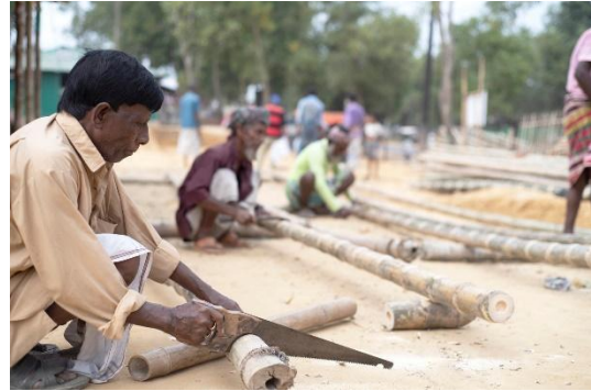
Gambar 13. Proses Kontruksi Ukhia School Sumber: Archdaily , 2020
