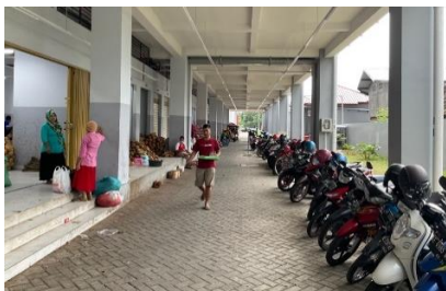
Figure 14. Drainage system area in the Legi Market area
