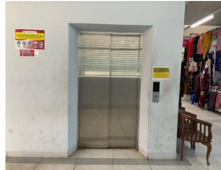
Figure 7. Elevator Facility at Legi Market Source: Personal Documentation, 2022.
