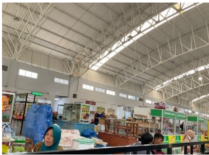
Figure 13. Natural ventilation in building at Legi Market
