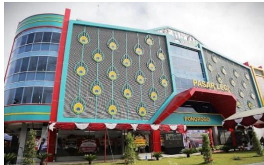
Figure 1. Legi Market Building
