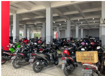
Figure 6. Condition of parking area facilities at Legi Market Source: Personal Documentation, 2022.
