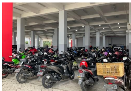
Figure 6. Condition of parking area facilities at Legi Market Source: Personal Documentation, 2022.
