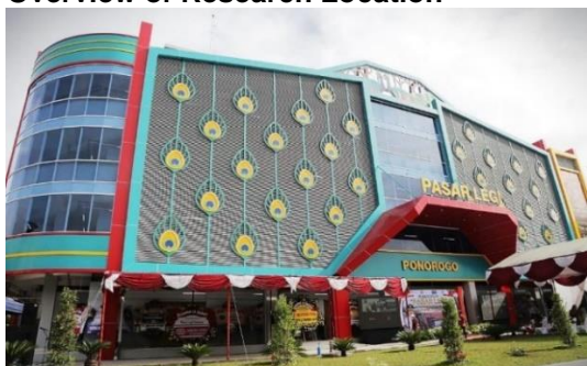
Figure 1. Legi Market Building
